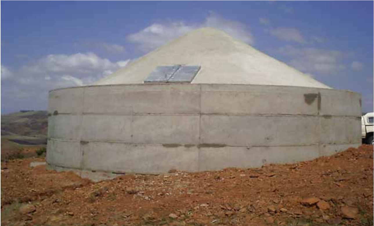
Reservoir constructed at Simdlangetsha west regional scheme
